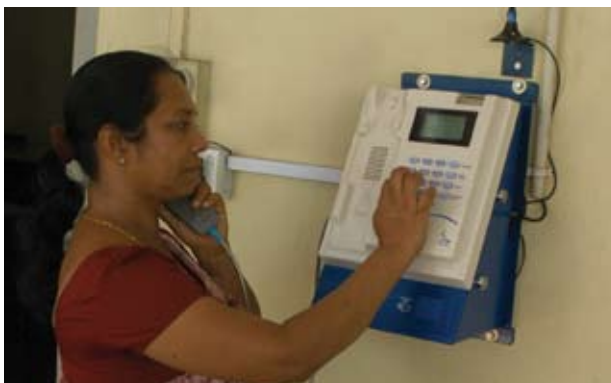
SLT's ubiquitous pay phone booths across the island were upgraded in the year under review
